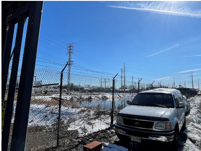
Rail yard infrastructure
