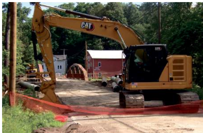
Photo by Pete Lindemann Construction is underway on the old bridge on Caverns Road by the Bramanville Grist Mill in Howes Cave.
